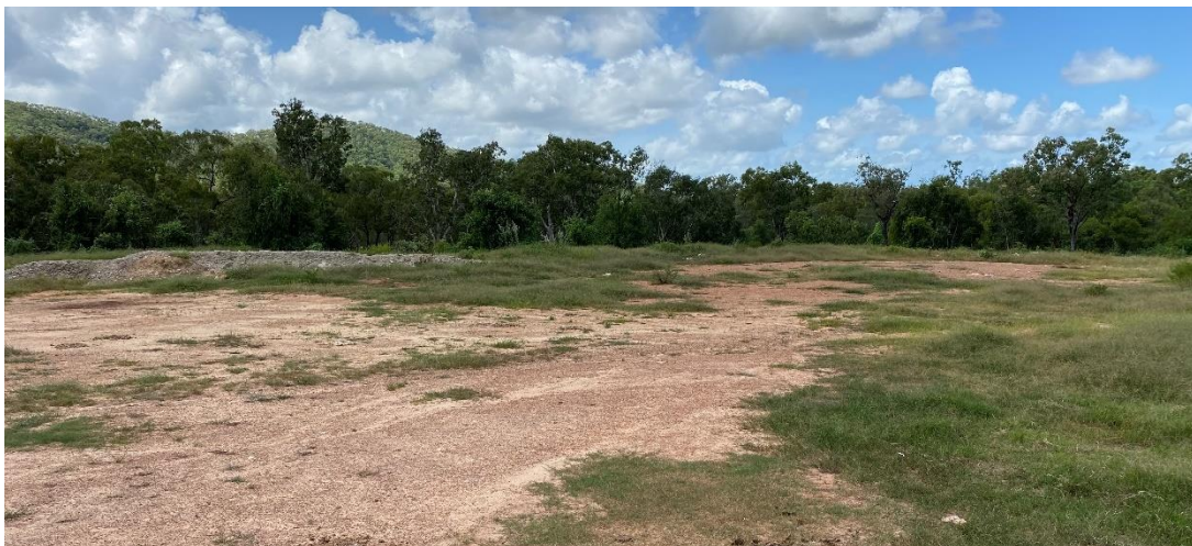
Image 8 Hope Vale landfill after significant earth works
