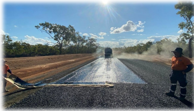
Bitumen resealing in the region.
