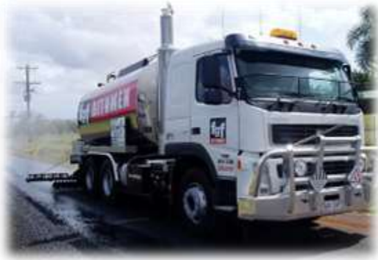
Figure 9 Bitumen Resealing by fgf Bitumen Crew
