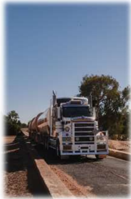
Figure 4 Road Train on Gilbert River Bridge
