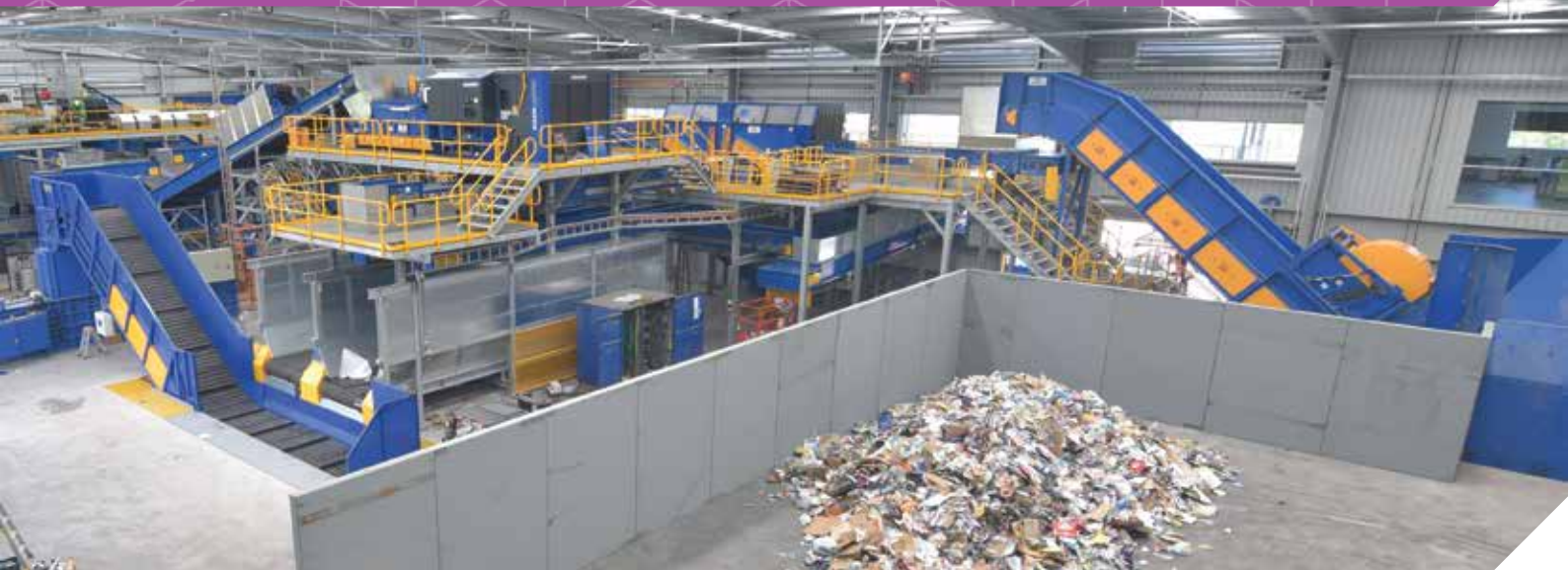
Cairns material Recovery Facility, Design and Construction by RDT.
