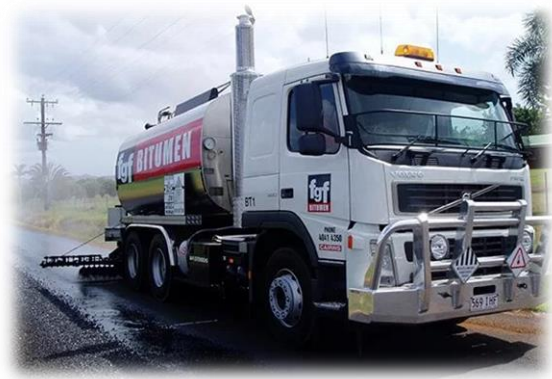
Bitumen Resealing by fgj Bitumen crew
