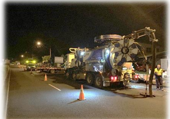
Figure 5- Works on sewers at night are sometimes required for high-flow sewers to minimise disruption to residents.
