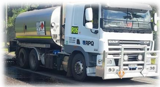
Figure 3 - Bitumen Resealing at Cassowary Coast Regional Council
