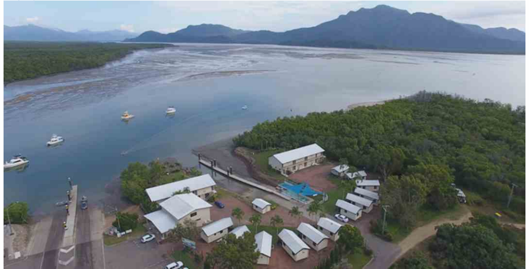
Figure 7: The Dungeness Facility.
