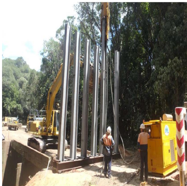
Figure 4- Maunder Ck - Driving Steel Piling
